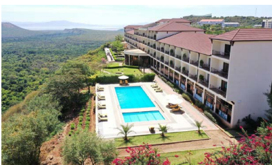
ARBA MINCH: HOTEL HAILE RESORT
