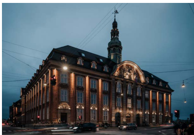
COPENHAGUE: HOTEL VILLA COPENHAGUEN
